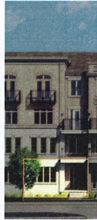
Typical Rear Elevation - Partial
